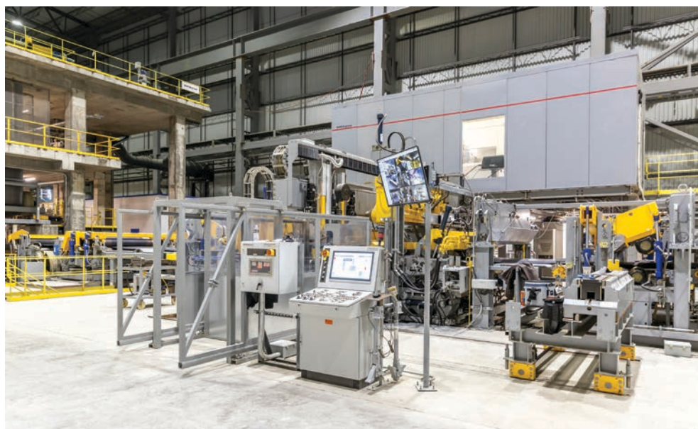
FIGURE 7. The X-Pro laser welder is integrated in the new pickling line/tandem cold mill at Big River Steel.
